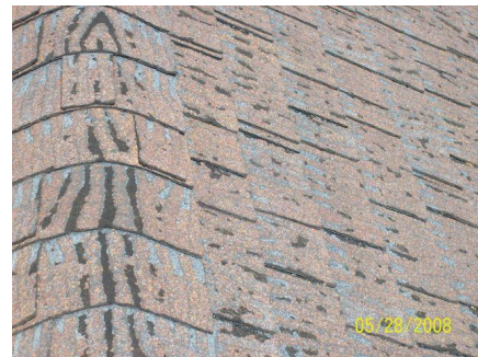
Observed large-scale surface damage at shingles, especially south and west-facing
