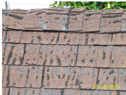
Observed large-scale surface damage at shingles, especially south and west-facing
